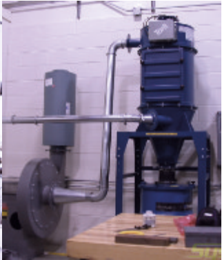
VACUUM LEAK DETECTION
