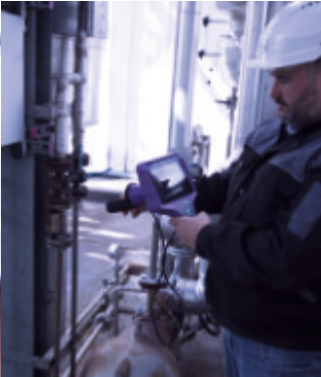
STEAM TRAP INSPECTION
